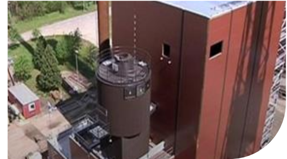
First demonstration scale integrated pyrolysis unit, Fortum
