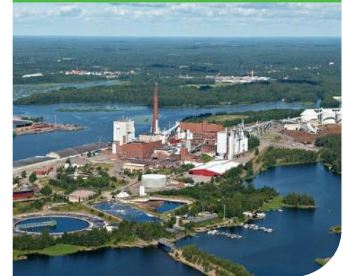
Stora Enso Sunila, Kotka, Finland
