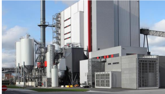
Valmet's CYMIC boiler at Stora Enso Langerbrugge
